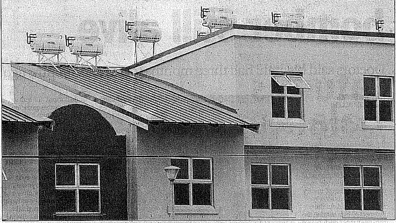
SOLAR POWER: The roofs of the new eco-friendly housing project in Steenberg sport scores of solar panels and solar geysers. The first 450 units of the project are ready for tenants. PICTURE: BRENTON GEACH
